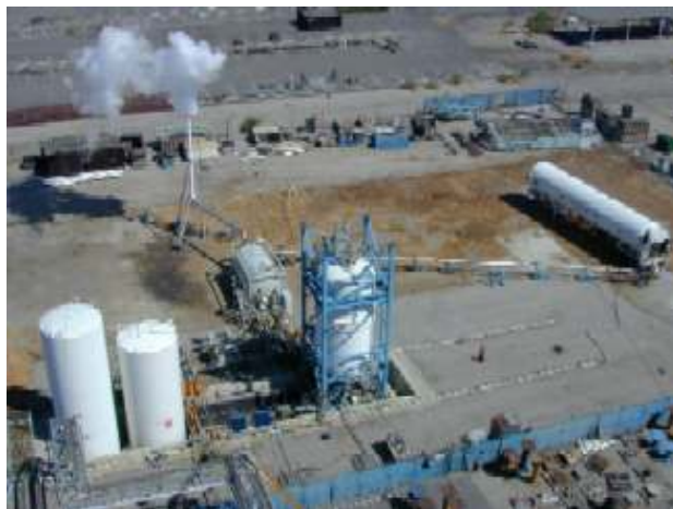
Figure 4. Large Scale Densification Test Bed
